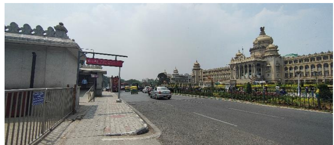
Fig. 4 Ramps at the entry points of the metro station
