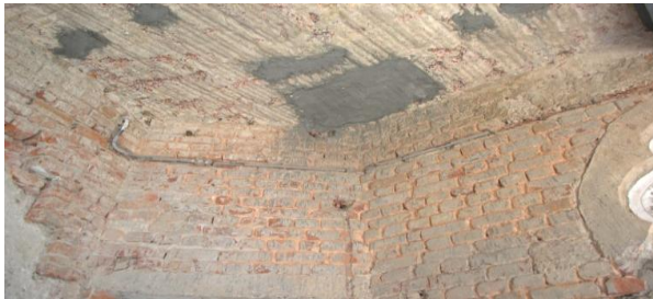
Fig.6. Apply of pre packed polymer modified protective mortar
