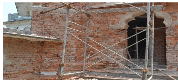
Fig.5. Removal of existing plaster
