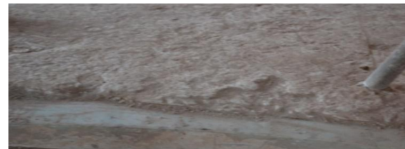
Fig.4. Layer of plaster of Paris over the floor
