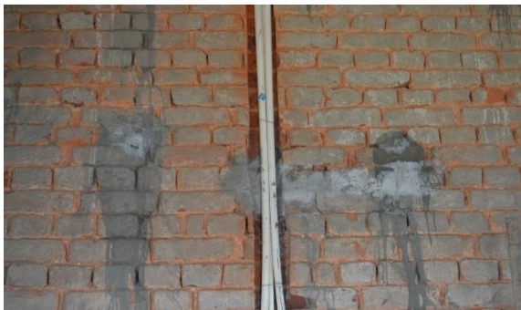
Fig.7. Injection of chemical (epoxy base)
