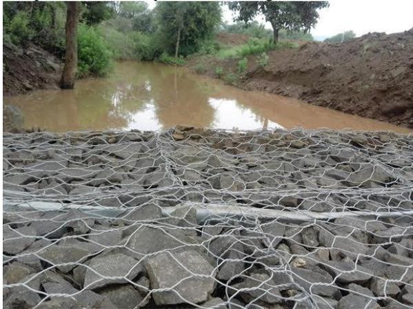
Fig. 4: Gabion Structures
