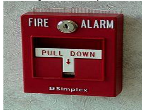
Fig. 2 : Pull Alarm System
