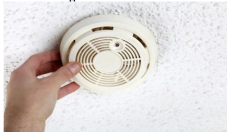
Fig. 1: Smoke detector
