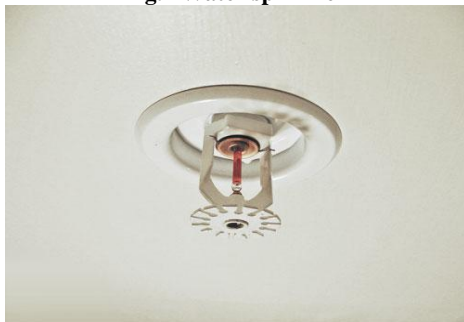
Fig. 2 Water sprinkler
