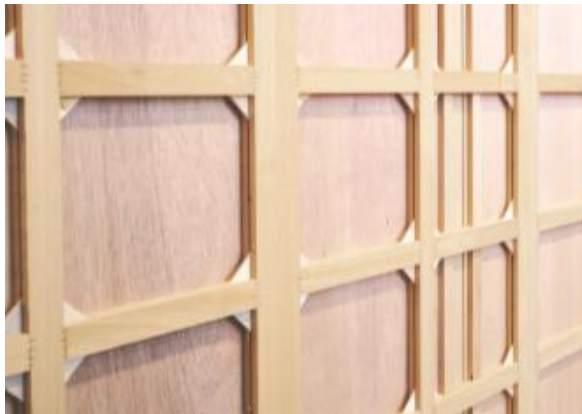
Fig 5: Wall carcass in mock-up, taken by author
