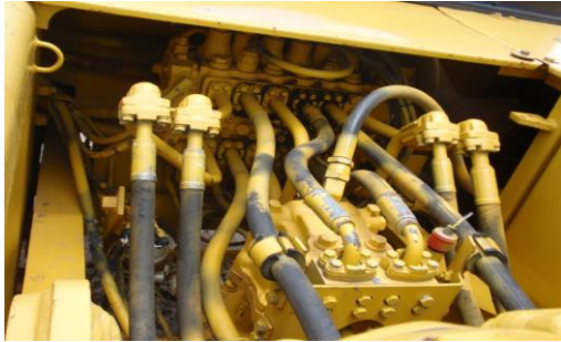
Fig.7: Hydraulic Block with hoses to control the cylinders and other operations
