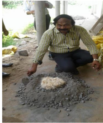
Mixing of concrete with banana fibres
