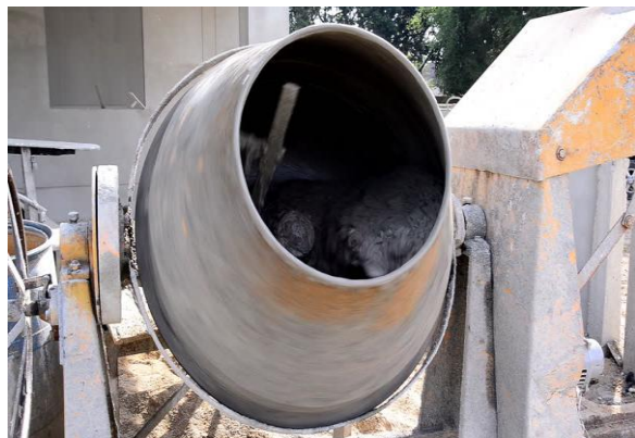
Figure 7.1: site view of mixer machine
