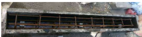
Fig 2: Fixing of reinforcement with cover inside the mould
