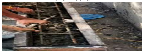
Fig 2: Fixing of reinforcement with cover inside the mould
