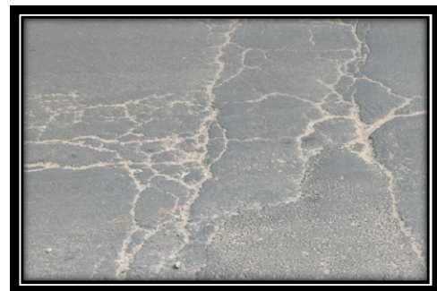
Fig 1: Alligator cracking
