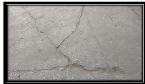
Fig 2: Block Cracking
