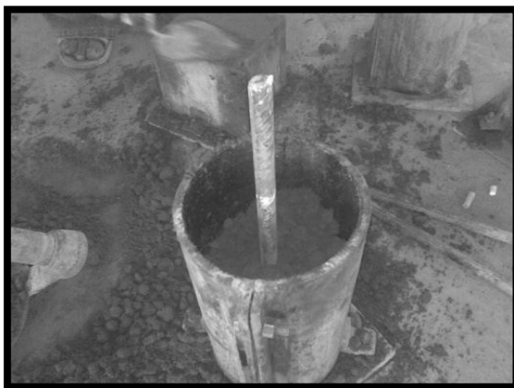
Figure – 7 placing of reinforcement
