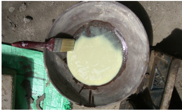
Fig 2: Mixing of bonding chemical [Base + Hardener]
