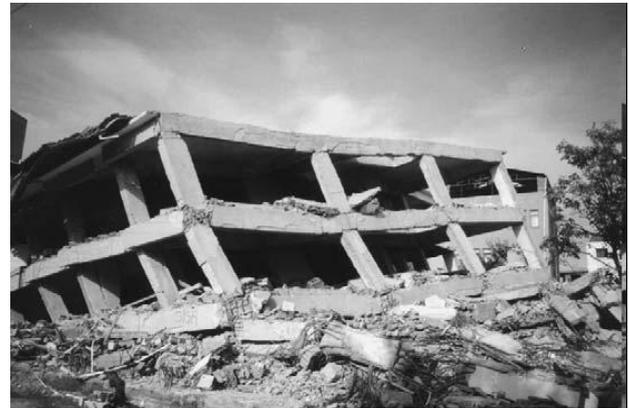
**Figure 1 Collapsed Reinforced Concrete Structure during Kocaeli Earthquake (Reference: [www.thecivilbuilders.com](http://www.thecivilbuilders.com))**
