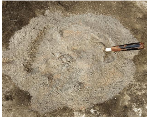
Fig.1. Mixing of ECC concrete.
