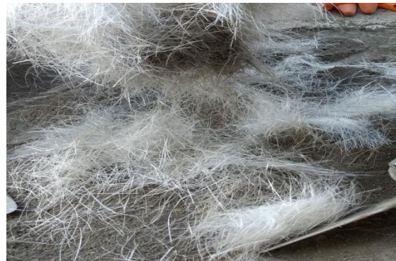
Fig.1.1 Mixing of PVA Fibre in Concrete.
