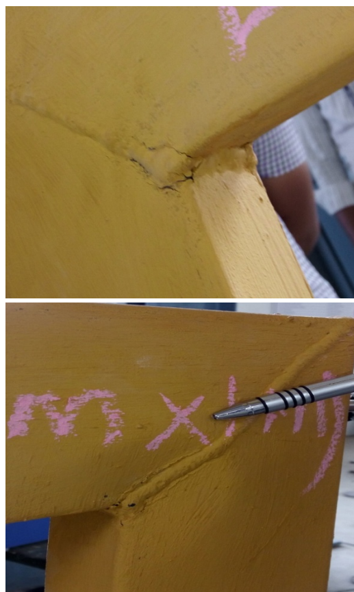
Figure 8. Failure of bare frame
