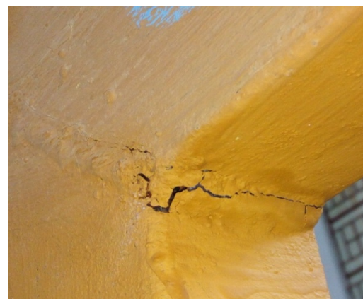
Figure 6: Failure of composite frame
