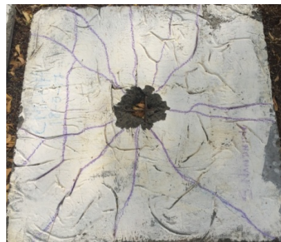
Figure 10 Crack pattern of CM-HF
