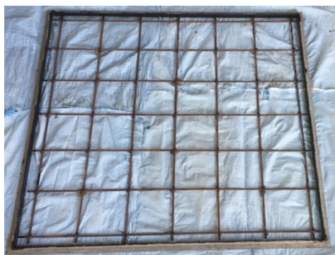
Figure 2 Reinforcement used in slab
