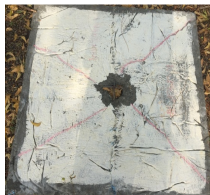
Figure 11 Crack pattern of 10SFLPMP-HF
