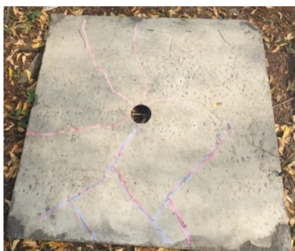
Figure 8 Crack pattern of CM
