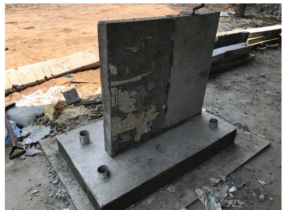
Fig 10: Erected wall panels
