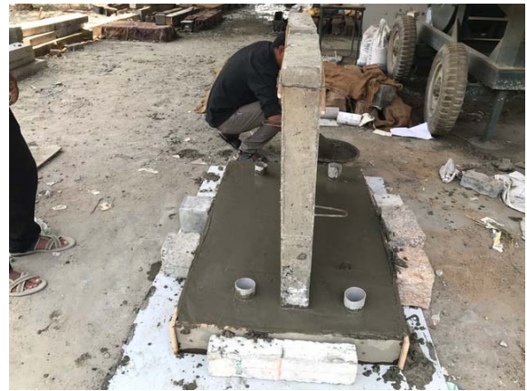
Fig 9 : Casting of wall panel and slab
