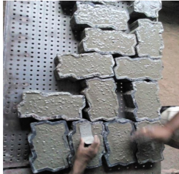
Fig.2 Compaction using Table Vibrator
