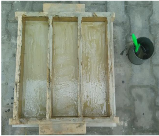
Fig 4: Mould oiled before casting of thickness 20 mm
