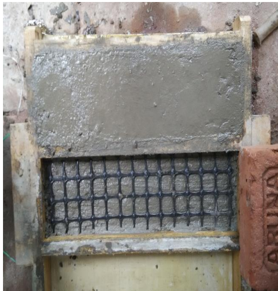
Fig 5: Placing of layers in mortar
