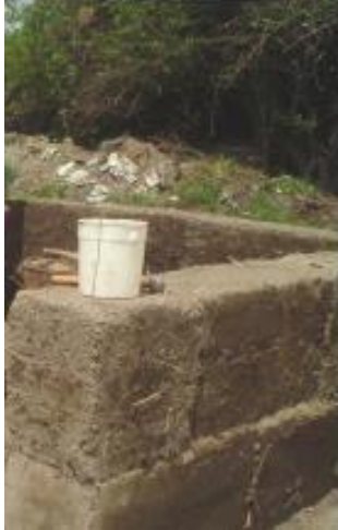
Fig. 2 Typical construction process of rammed earth walls (Adolfo Preciado and Juan Carlos Santos, 2020) [16]
