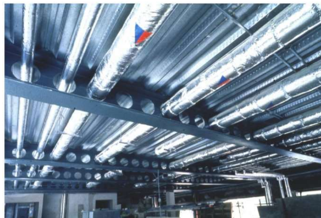
Fig. 1 Passing Pipes Through a Beam With an Opening Web [3].
