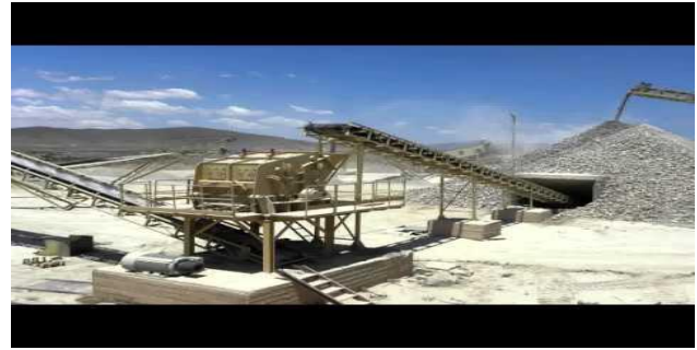
(1.8) Secondary Stage of Stone Crushing
