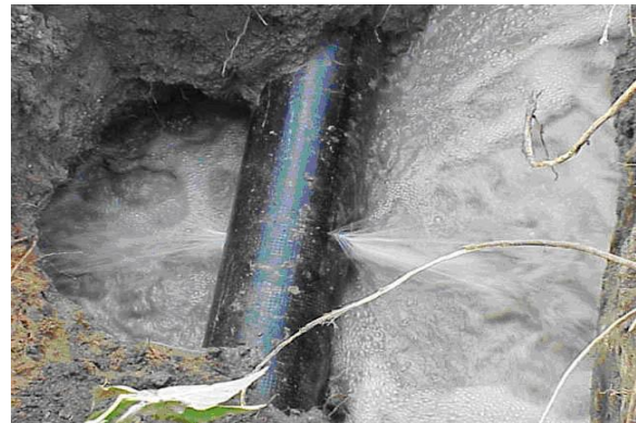
Figure 2.2 Component of Real Loss- Leakages
