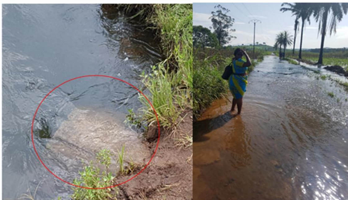
Fig. 14. Submerged nozzle and the main road covered with water
