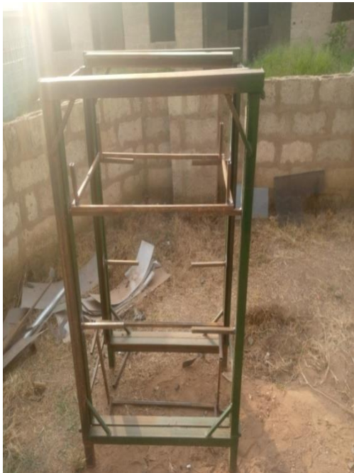
Plate 1a. Construction of a rectangle ECS
