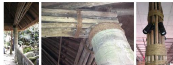
Fig 4.2 Examples of Timber Construction Detail
