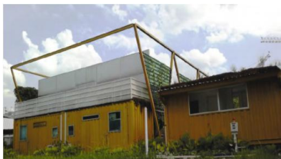
Fig 4.3 Re-using of shipping containers in new buildings
