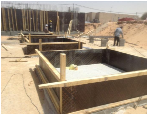
Figure 3 Isolated footing in practical
