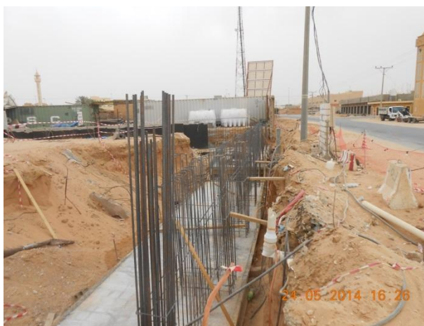
Figure 6 Raft footing in practical
