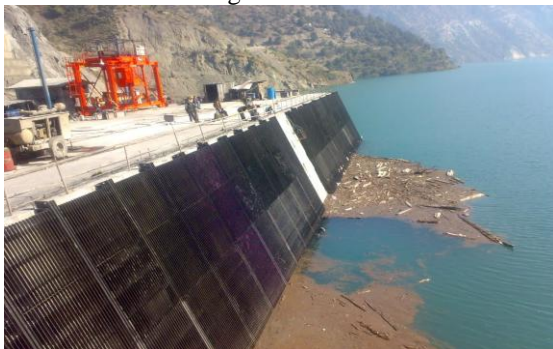
Figure 2 (The intake structure of BHEP)
