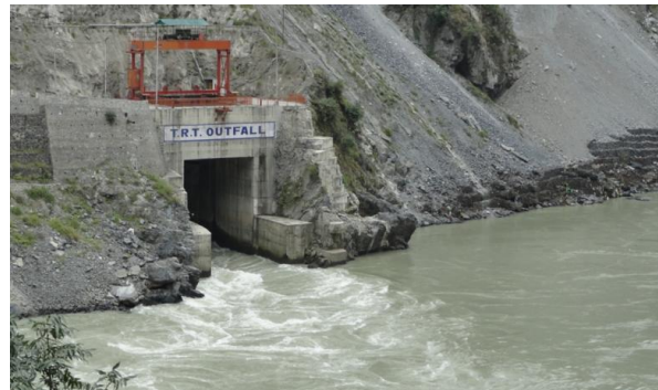
Figure 7 (TRT Outfall of Stage-I of BHEP)
