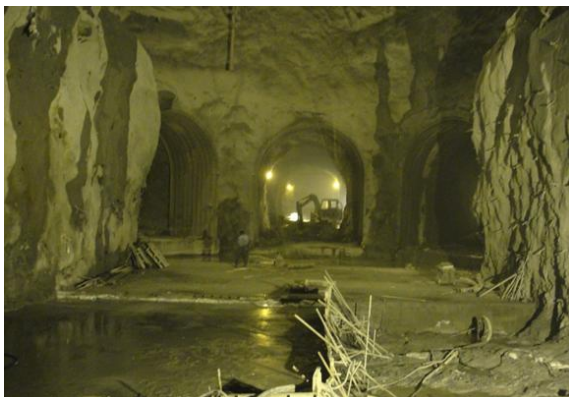
Figure 5 (Surge chamber from where HRT will differentiate into 3 Penstocks)
