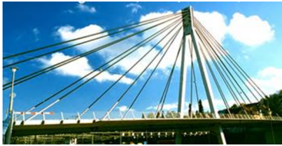
Figure 6: Stock-bridge with CFRP cables.”SOURCE: Meier [23]”
