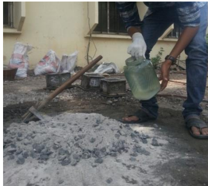
Photo 3: - During Adding Of Geopolymer In Dry Concrete
