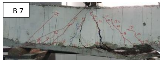
Fig. 8 Failure Cracks For Strengthened Beams B6 & B7
