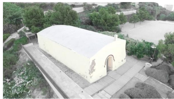
Fig. 3: Image of the Polvorín De La Ereta Made with Dron at a Height of 20 Meters above the Ground Level
