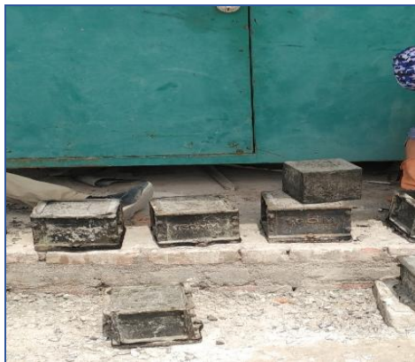
Fig 5. De-moulding of Cubes
