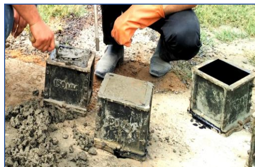
Fig 3. Casting of Cubes
