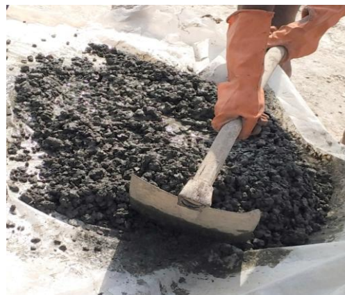
Fig 2. Mixing of Concrete
