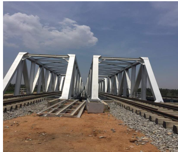
Figure 2: Two Lane Steel Railway Bridge
