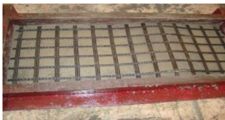
Fig.5 Placing of Geogrid Mesh
