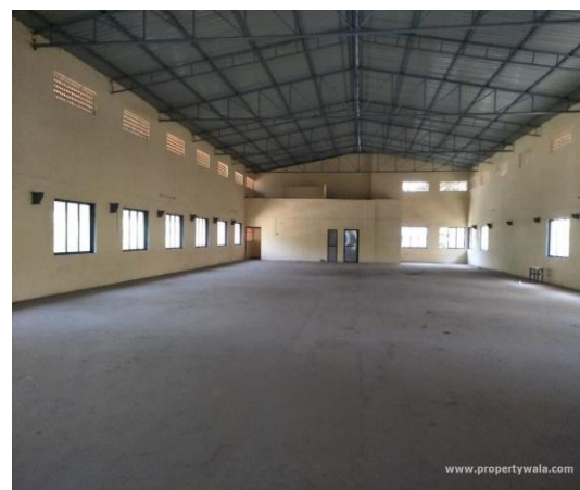
Fig. 12: internal view of an industrial building
