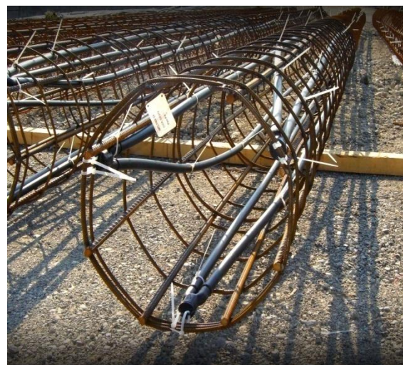
Fig1: Energy Piles structure
