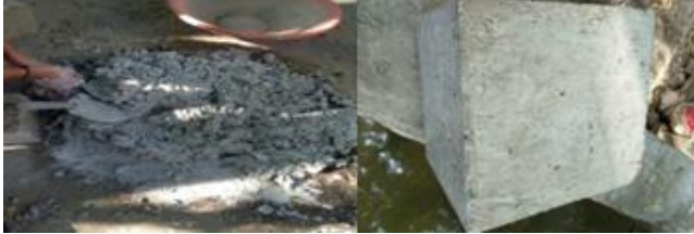
Fig 4 CONCRETE CASTING AND CURING
