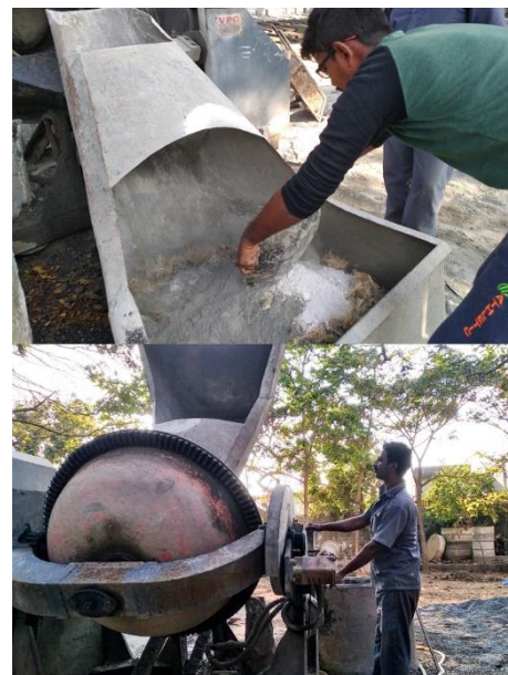
Fig 7: Batching and Mixing
