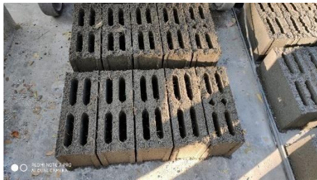
Fig 8: Casting of blocks
