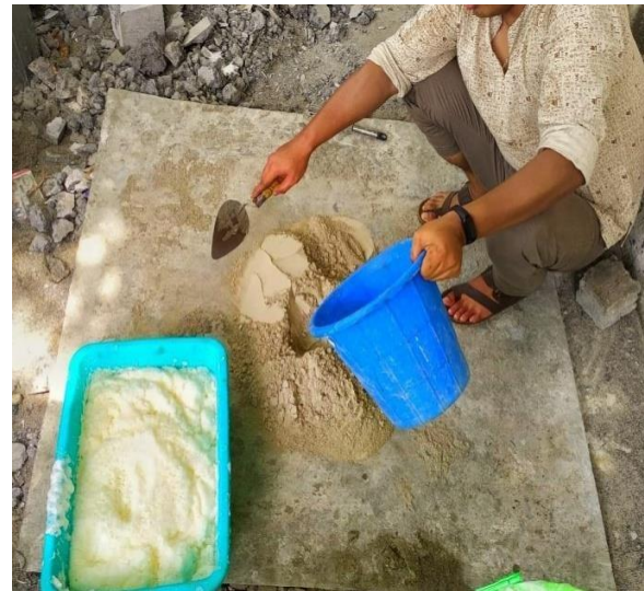
Fig 1: Mixing of foamed geopolymer concrete
