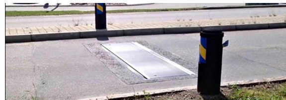
Fig. 10 Acti-bump anti-speeding system on the road
