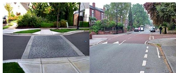
Fig. 5 Flat-topped midblock calming extended speed hump
