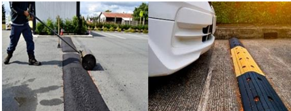
Fig. 1 Speed bump preparation and installation in parking lots
