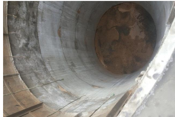
Photo 1 Off-site Pit Latrine [6]
