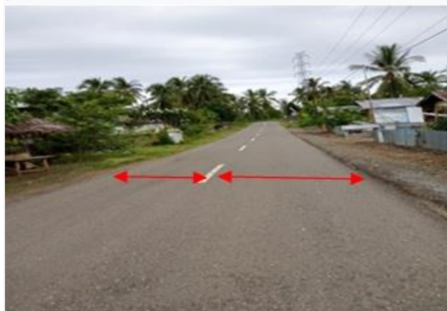
Figure 4. The width of the traffic lane is 2.4 m
