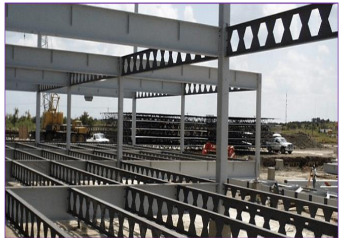
Fig. 1 High bay span castellated beam steel structure
