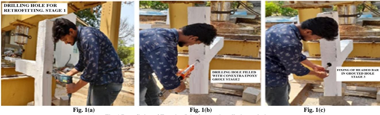
Fig. 1 Retrofitting of Exterior Joint by post installation technique
