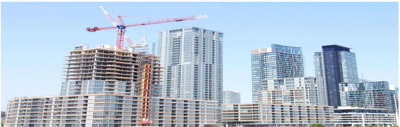
Fig. 1.1 Tower with podium structure
