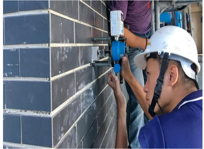
Fig. 3 Pull-out test for tiles (2)
