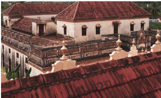
Fig. 10 Roofs and parapets in building facade - Chettinad house at Karaikudi, Tamilnadu
