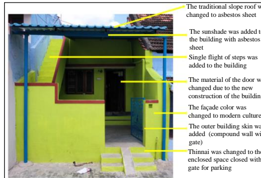
Fig. 37 Sample 8 house facade
