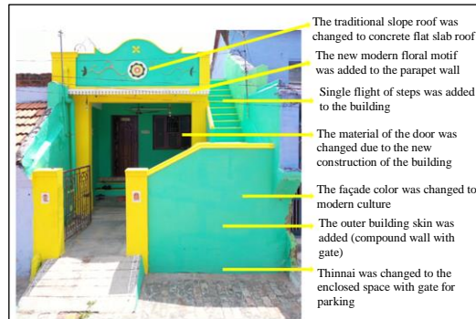
Fig. 39 Sample 10 house facade
