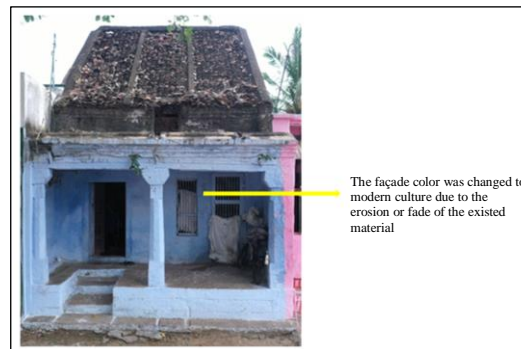
Fig. 45 Sample 16 house facade
