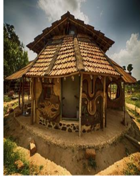
Fig. 8 Materials in building facade – Traditional mud house of South Tamilnadu
