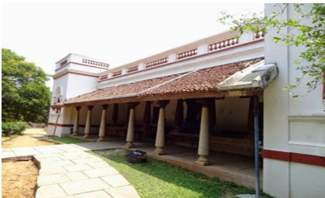
Fig. 11 Roofs and parapets in building facade – traditional homes from South Tamilnadu
