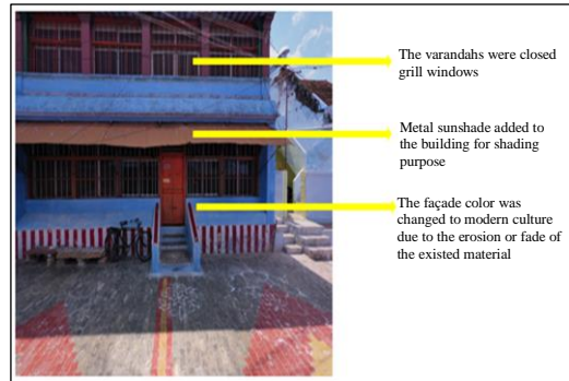
Fig. 42 Sample 13 house facade
