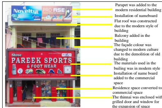
Fig. 51 Sample 22 house facade
