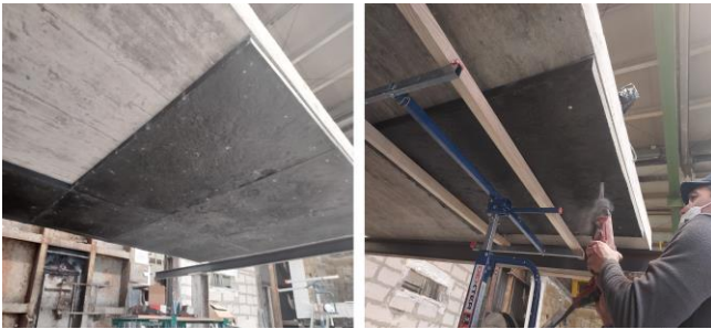
Fig. 8 Precast sample installation of the fire resistance test for the protection of concrete structural members
