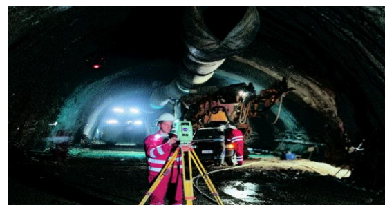
Fig. 3 Geodetic work to determine the blasting, center, elevation, and contour of the tunnel cross-section
