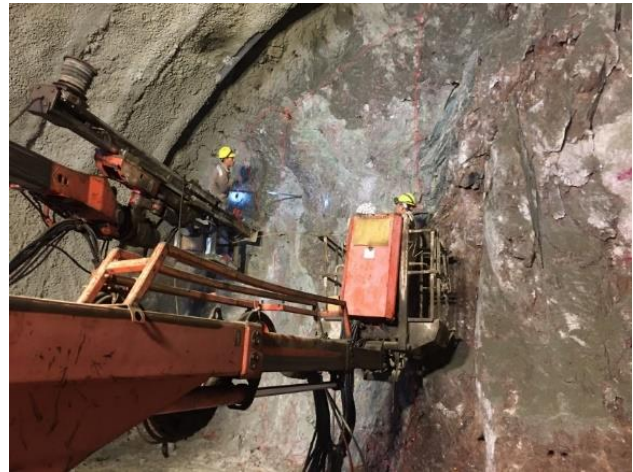
Fig. 5 Work of loading drugs into holes drilled on the tunnel face
