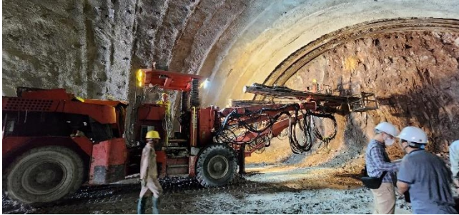
Fig. 4 Drilling of tunnel face blasting holes using self-propelled drilling vehicles
